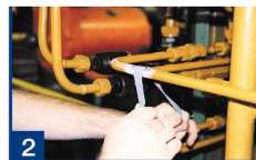
remove paint and clean pipe
