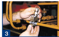
clamp SC onto pipe
